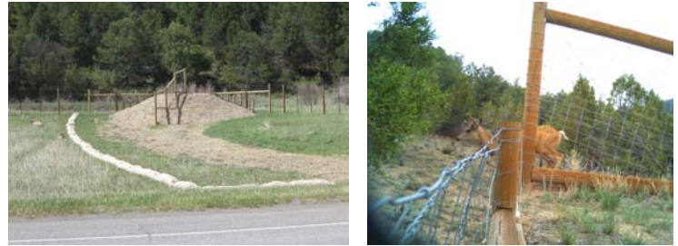
Wildlife escape ramps, like the examples above, allow trapped animals safe passage out of the highway ROW.
